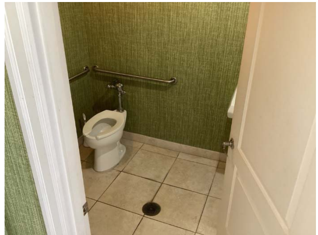
Rest room overview
