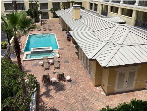
Paver pool deck overview
