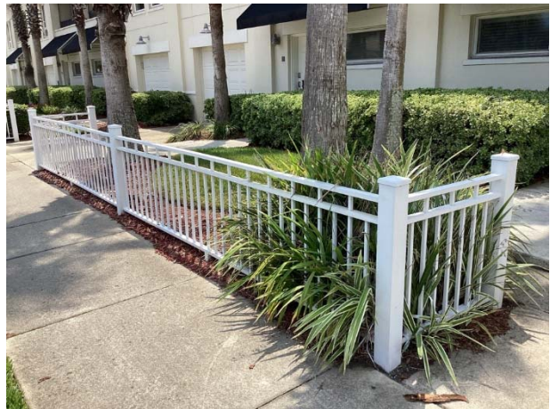
Aluminum railings at rear of building.
