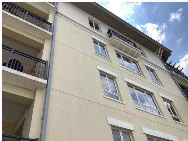
Stucco wall finishes
