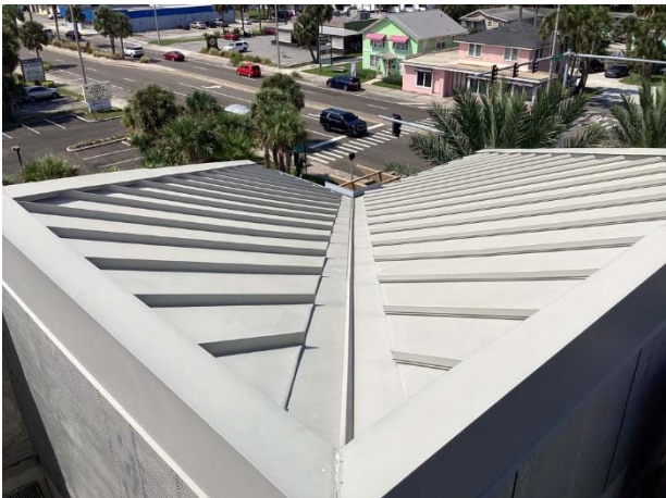
Roof valley view
