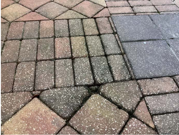
Spalled pavers
