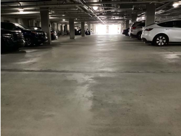
On-grade garage floor overview
