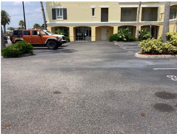
Asphalt pavement parking lot overview
