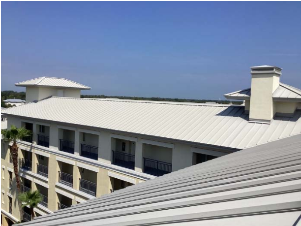
Metal roofs overview
