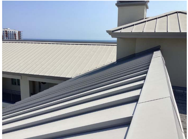
Standing seam metal roof
