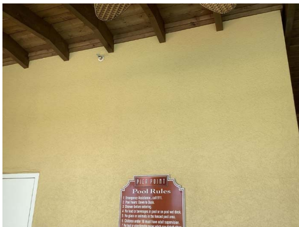
Stucco at pool rest room exterior
