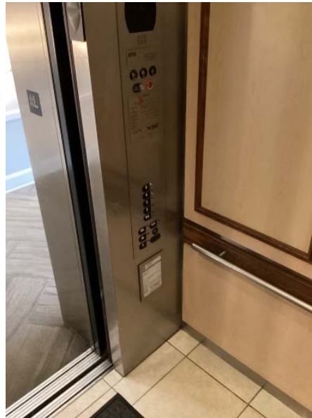
Elevator cab finishes
