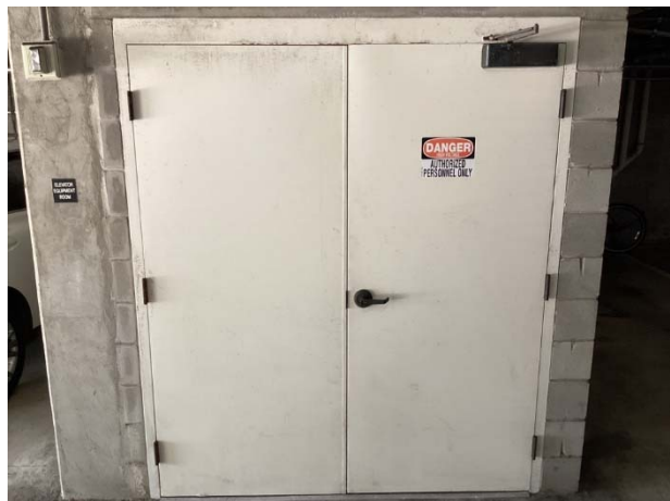
Electrical room doors
