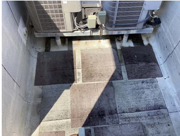
Lower modified bitumen roof
