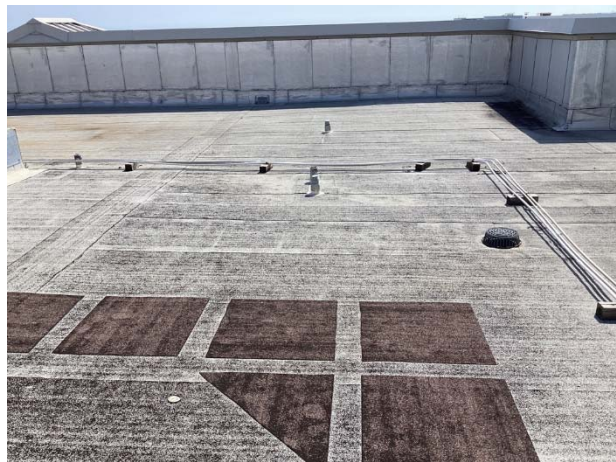
Modified bitumen roof overview
