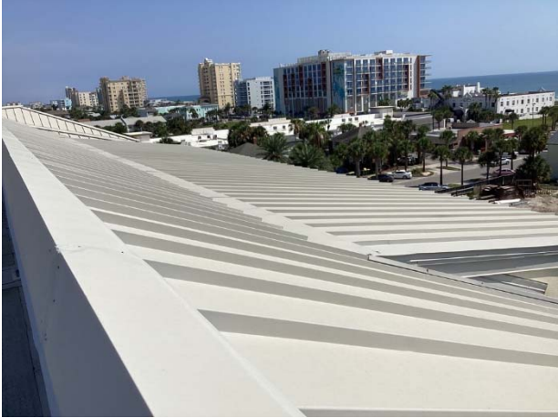
Metal roofs overview
