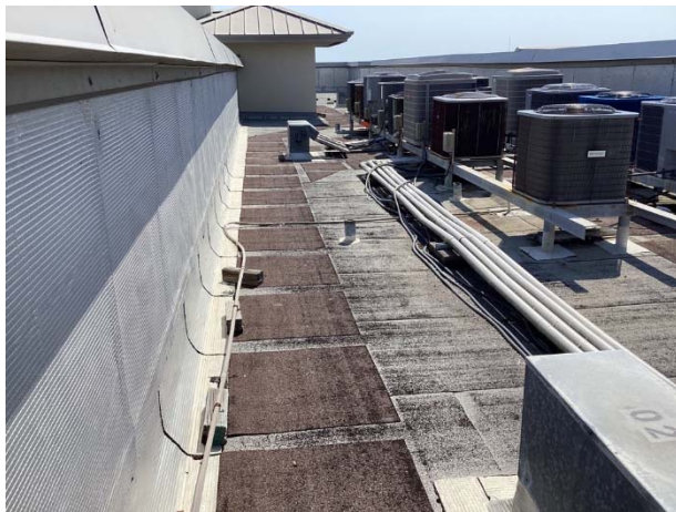
Modified bitumen roof overview
