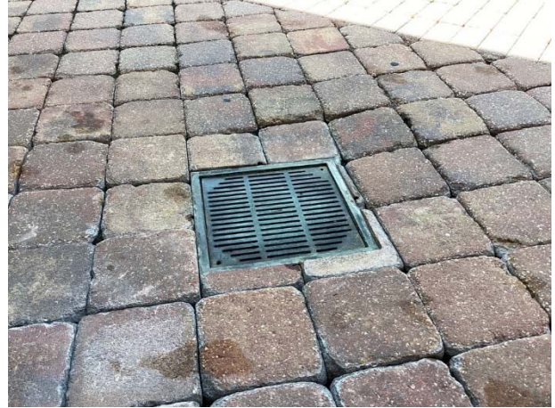
Pavers deck drain
