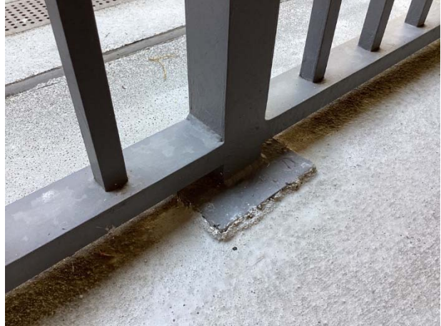
Mechanically attached railing post
