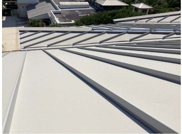
Standing seam metal roof
