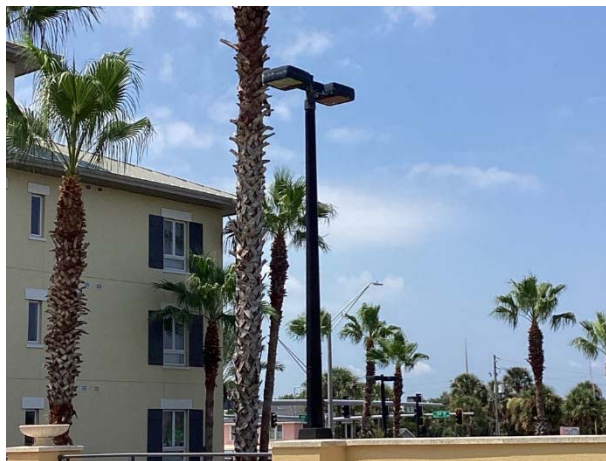
Light pole and fixtures
