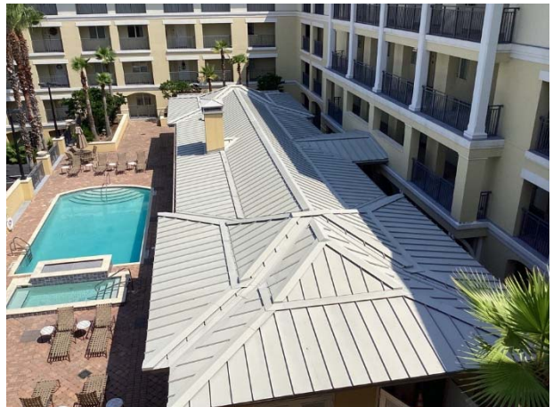
Club room roof overview
