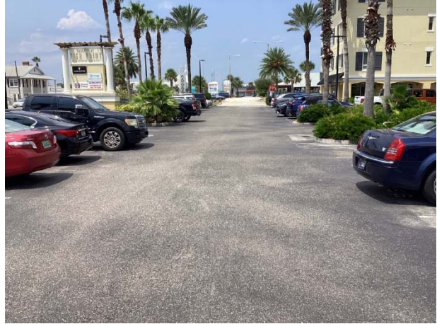
Asphalt pavement parking lot overview
