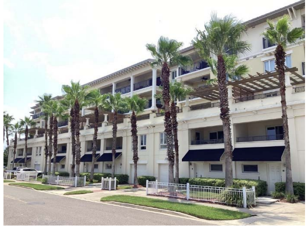
Terraces at rear of building
