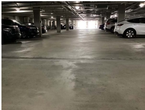
On-grade garage floor overview
