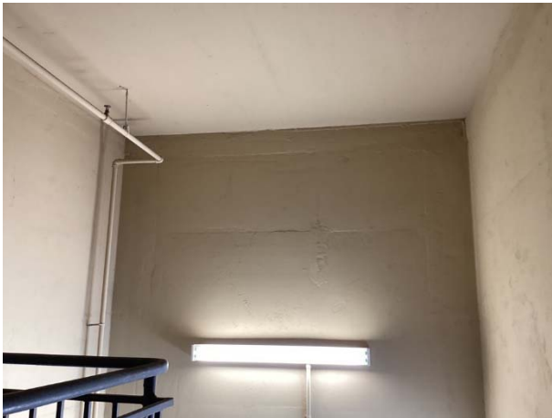
Stairwell paint finishes
